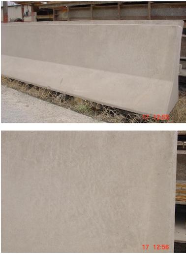
**Fig. 12: Form Finish of Road Barrier Unit**
