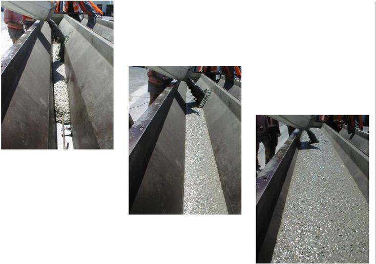
**Fig. 11: Casting SCC in Road Barrier Unit**
